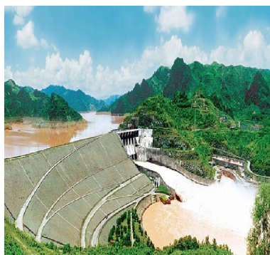
(b) Hoa Binh Dam and Hydroelectricity Plant
